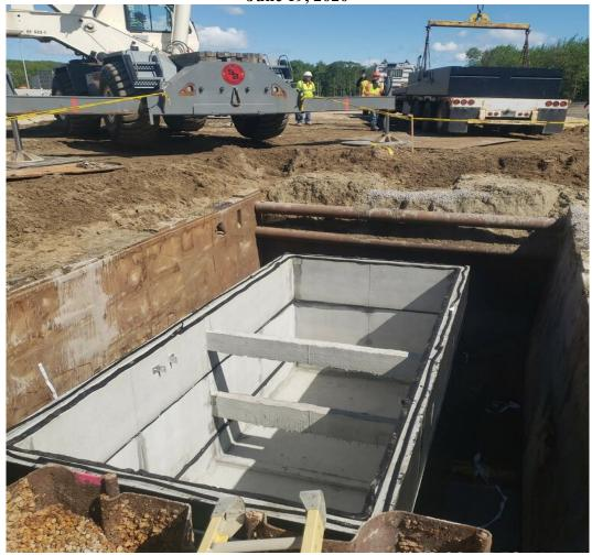
This crane is about to set the cover on the oil and water separator at the NB plaza.
