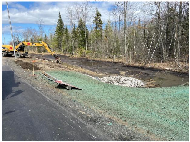
An excavator grades the ditch and inslope at the NB Kennebunk on ramp.
