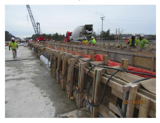
The parapet wall in the foreground shows the heater hoses draped over the fresh concrete prior to the weepers hoses being turned on and insulated blankets pulled over the forms.
