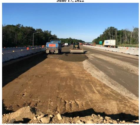
Looking south in the median, Sargent crews are installing and prepping gravel for new permanent median concrete barrier.
