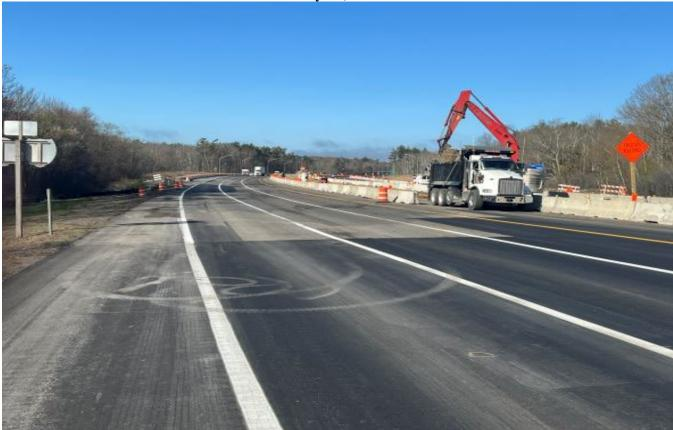
Looking south from the northbound lane, Sargent crews are excavating for new drainage during the day while milling and paving mainline at night.
