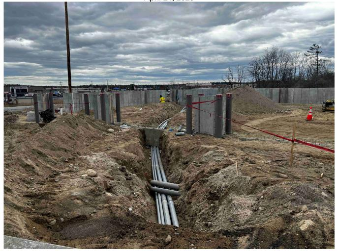
An electrician is working on conduits that will be covered by pavement and the concrete slab once the project is complete.
