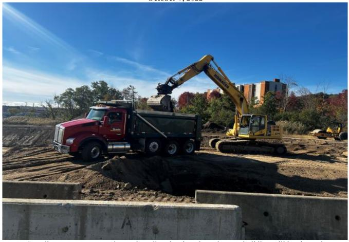
Grondin crews are excavating and grading the site where the new building will be situated.
