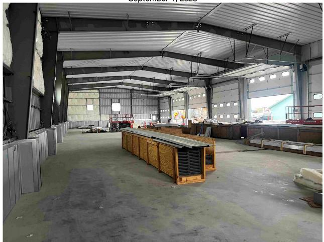
Looking west inside the new Crosby building. Notice the insulation on the far wall and the recently installed ceiling panels.
