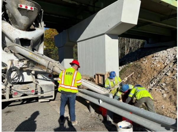
North bound Bennett Road concrete repairs. CPM crews are placing concrete into the forms.
