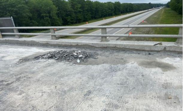
Bennett Road looking north.The concrete deck was in poor condition along the gutter lines.Contractor:CPM ConstructorsBid Amount: \$1,298,652.20Percent Complete last approved pay estimate:14.4 %
