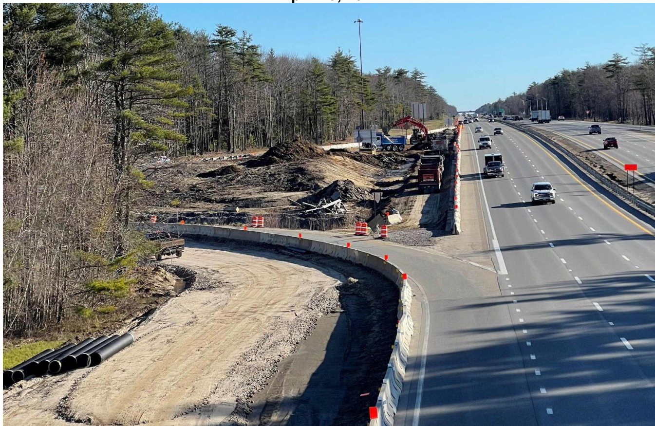
Looking north at the construction of the collector-distributor roadway at Exit 36.
