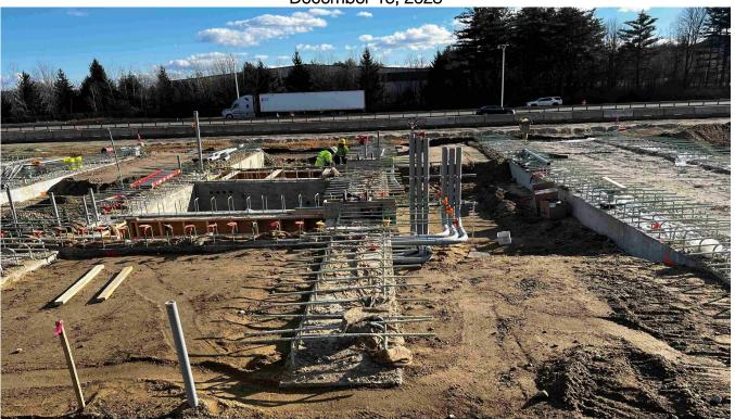
Southbound administration building foundation work is ongoing. Crews prepping for the concrete slab.
