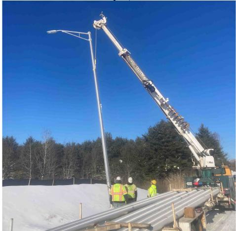
Looking northbound at Exit 36 departing, Moulison Heavy Electrical is standing light poles for the realigned off ramp.
