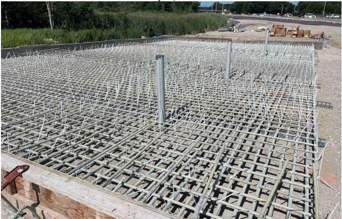
Looking north at the Exit 35 southbound departing slab, showing the Glass Fiber Reinforced Polymer mat. Contractor: Sargent Corporation Bid Amount: \$41,922,810.00
