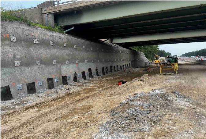
Looking north at the Exit 36 bridge, crews are making great progress on the soil nail wall.
