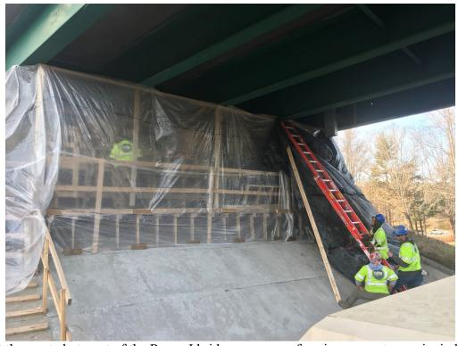
Looking at the west abutment of the Ramp J bridge: crews performing concrete repairs in heated tent.
