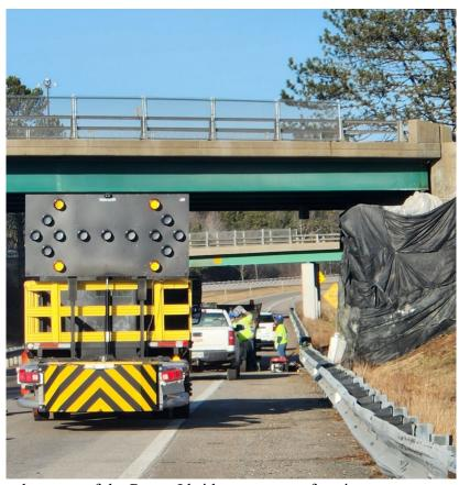
Looking at the east abutment of the Ramp J bridge: crews performing concrete repairs in heated tent.
