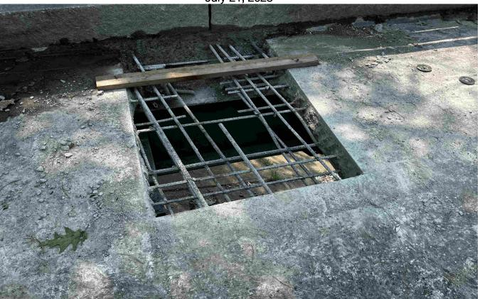
Ongoing full depth deck repairs around the new bridge drain along the southeast corner of Wilson Road Bridge.
