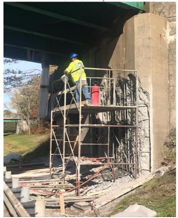
Looking at the east abutment of the Ramp J bridge: crews performing concrete repairs.
