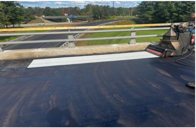
Looking north on the Ramp J bridge: crews are installing the high performance membrane.
