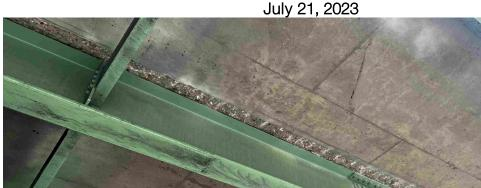
Concrete haunches were removed along the underside of Leighton Road, in Falmouth.
