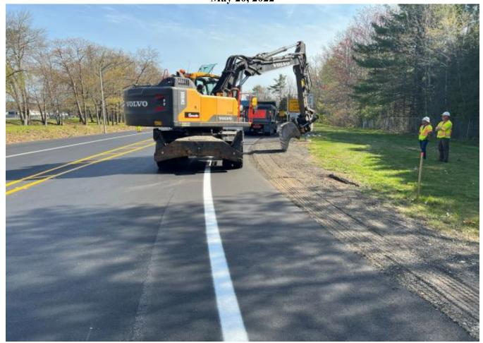
Grondin's excavator is backing up new pavement with reclaimed asphalt at the Exit 25 northbound plaza.
