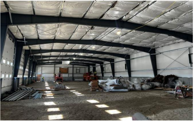
Looking west inside the new 8 bay garage. Crews are working on the ceiling insulation.
