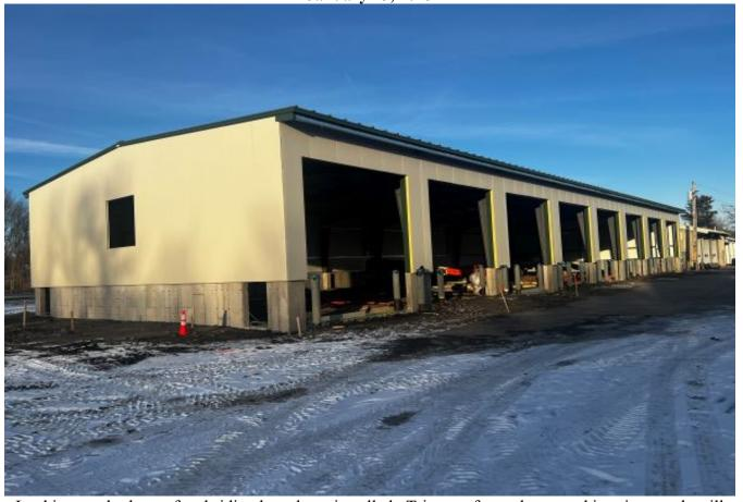
Looking north, the roof and siding have been installed. Trim, roof cap, doors, and interior panels will continue to be installed this winter.
