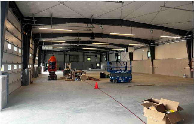
An electrician is working on the wiring for the overhead doors. Note that the new LED lighting is operational on temporary power.
