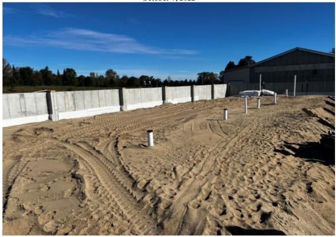
Looking north at the inside of the new building. The white pipes are stubs for interior drains.
