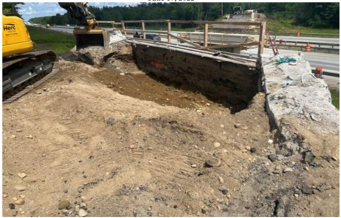
Looking east, the contractor is excavating behind the southbound abutment so crews can modify and repair the approach for the new bridge.
