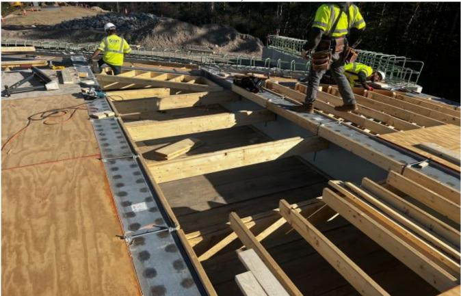
Looking east at the Scott Construction crew working on building the formwork for the bridge deck.
