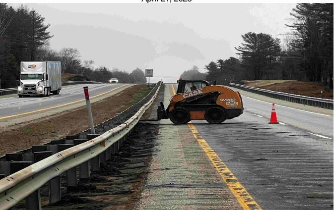
Looking north, a skid steer pushes built up material out from under the guard rail so an excavator can load it into a dump truck.
