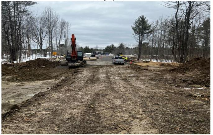
Looking towards Route 126, crews are grading subgrade and installing Type D gravel.
