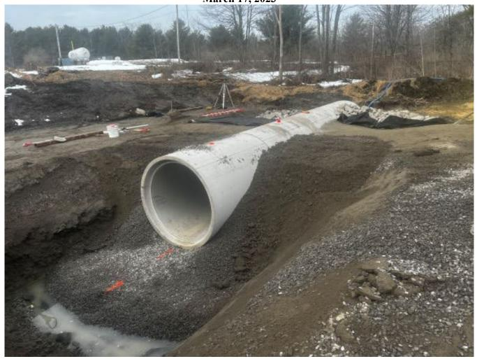
Looking southwest at the 60" reinforced concrete pipe being installed by Grondin crews along the new 102 on ramp.
