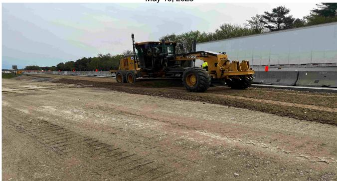
Looking north at the future gore and merge area, Grondin's grader is prepping the gravel for pavement.
