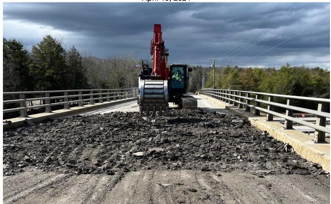
Looking west, an excavator is removing pavement prior to the deck being demolished.
