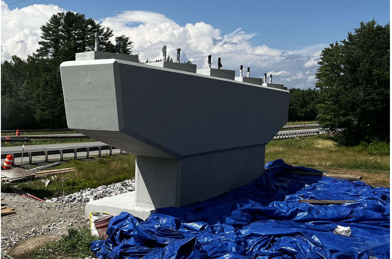
Looking north at the recently reconstructed eastern most pier.
