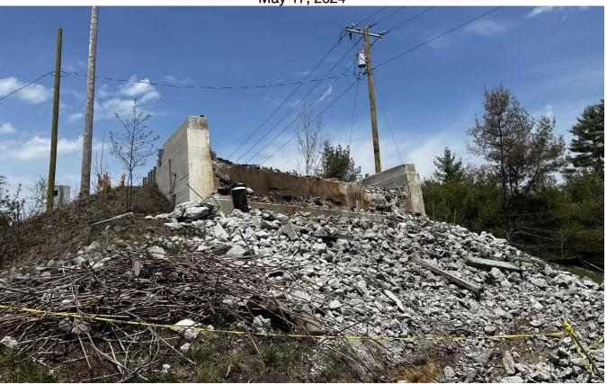
Looking west at the remains of the old bridge abutment prior to being rehabilitated.
