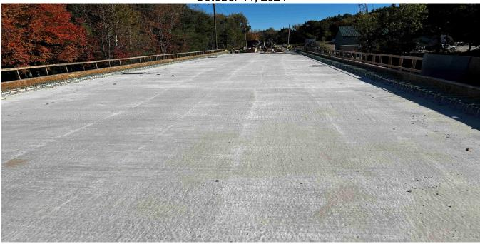
Looking east at the recently placed bridge deck. Crews will be placing the curbs in the next two weeks.
