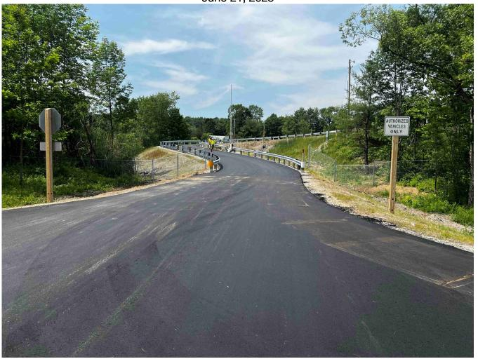
The Southbound EVR with surface pavement. Crews are touching up the loam and other incidentals prior to final completion.
