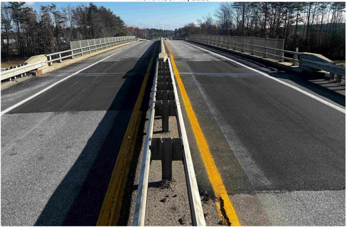
Looking east from the west approach, the repaired headers and pavement are in place.
