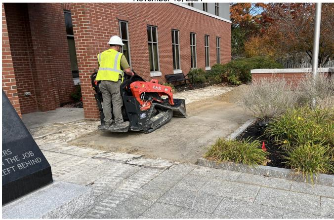
The contractor uses power equipment to remove damaged pavers from the walkway.
