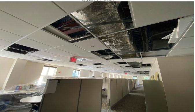
Electricians have removed ceiling tiles to make room for new LED lighting.
