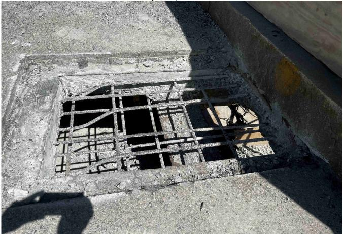
Concrete has been removed from the Spruce Creek bridge deck to facilitate the replacement of the rusted out bridge drain.
