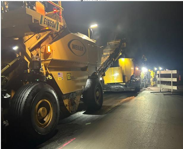
The transfer machine fills the hopper of the paver with hot mix asphalt. Contractor: Pike Industries, Inc. Bid Amount: \$18,302,432.00
