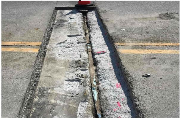
Looking at the eastern bridge joint on Route 35 in Kennebunk. Crews will rehab the concrete and replace the Asphaltic Plug Joint (APJ).
