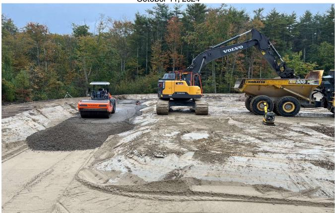
RJ Grondin is placing and compacting the structural fill for the foundation.
