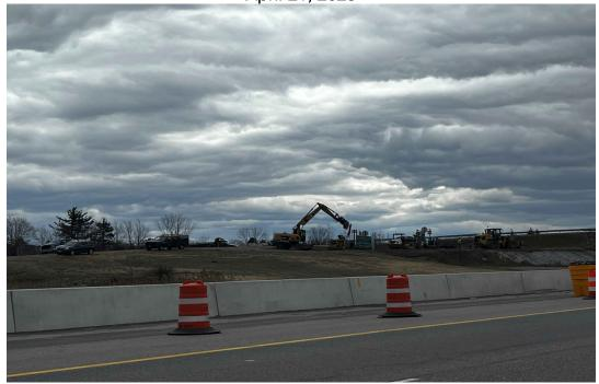
Shaw Brothers has their rubber tired excavator finish grading slopes adjacent to the new Exit 45 bridge.
