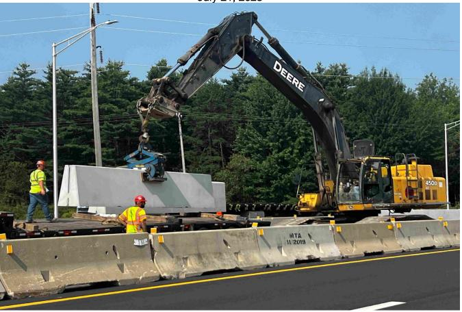
Looking west at one of the crews unloading median barrier for the Route 1 connector, just east of Maine Mall Road.
