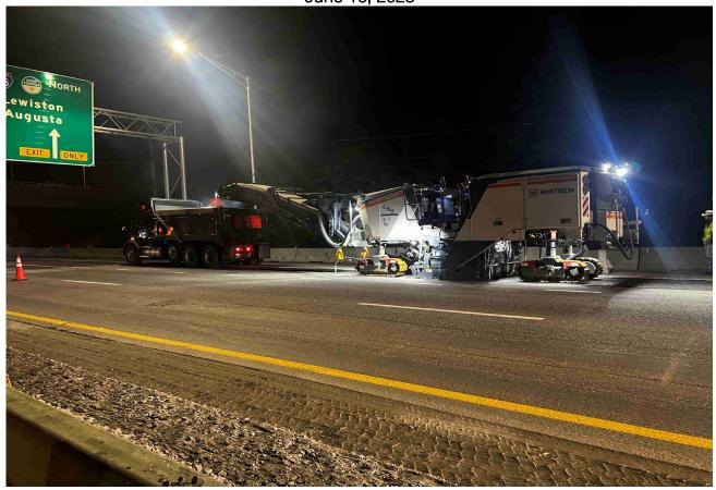
Heading west on the 703, a milling crew profiles the existing pavement to match modern highway standards and to improve drainage, and ride quality.
