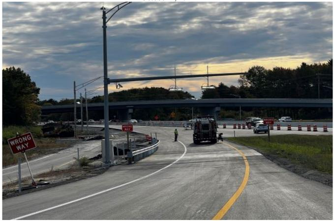
Looking south at the Exit 45 northbound exiting ramp, a paint truck stripes the newly constructed ramp.
