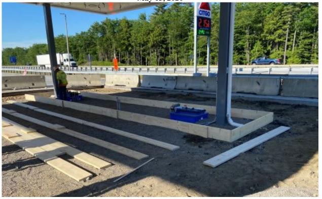
SRS crews are building concrete form work for the new gas dispensers in Gray.
