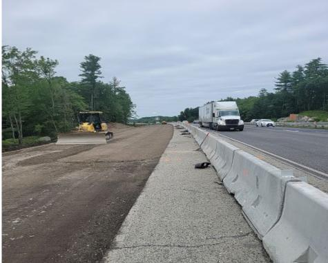
Looking north at exit 32, crews are finish grading gravel prior to base paving.Contractor:Pike Industries, Inc.Bid Amount: \$7,058,127.50
